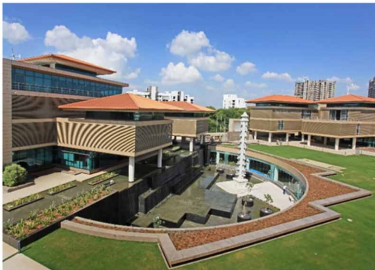
Figure 17. Suzlon One Earth (Pune, India) (Going Green, 2020)
