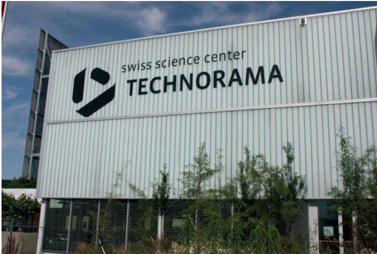
Figure 2: Park facade of the Technorama
