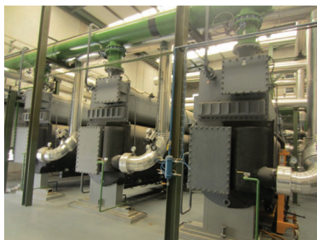
Figure 6: Absorption chillers at Geolit.
