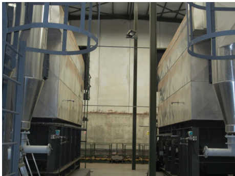
Figure 5: Biomass boilers (3,000 kW/boiler) at Geolit.
