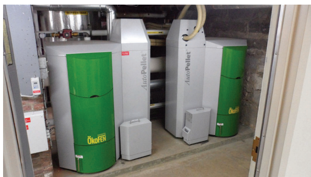
Figure 6: Two wood pellet boilers [12].
